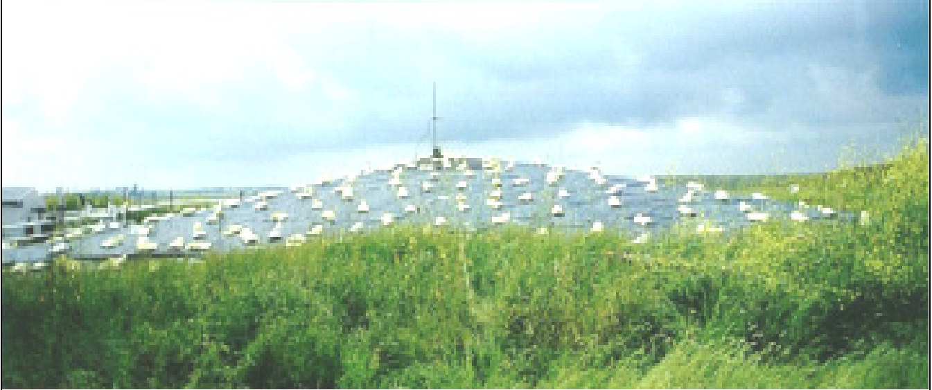
Landfill bioreactor cell, Yolo County, California
