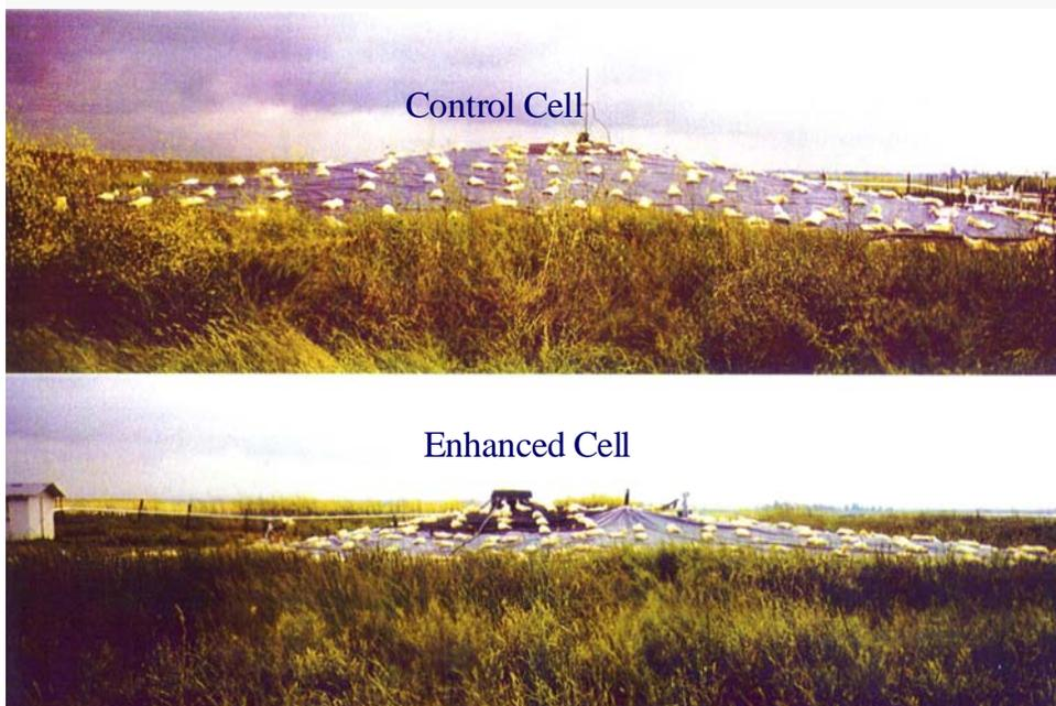
**Image 1. Surface profiles of the two 9,000-ton pilot cells operated 1995 to present. Note the waste volume loss indicated by the subsidence of the methane-enhanced cell. This subsidence is due to the destruction of organic waste solids (like paper fractions and food) to form landfill gas.**
