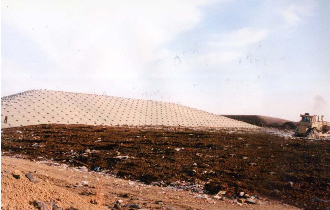
**Figure ES-2. Northeast cell, shortly after geomembrane coverage, is in the foreground. The northeast cell footprint is approximately 300 ft by 500 ft, and it contains 78,000 tons of methane-enhanced waste. The scale is also indicated by a person walking up the cell cover near the lower left corner of the cell.**
