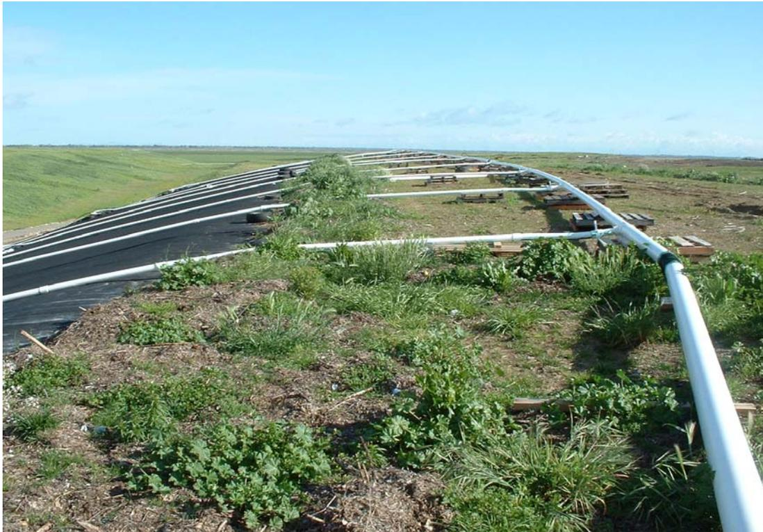
**Image 3. LFG collection lines connected to the main header on the west 6-acre cell.**
